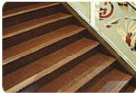
Steps within the center are fabricated from Imperial Red granite.
